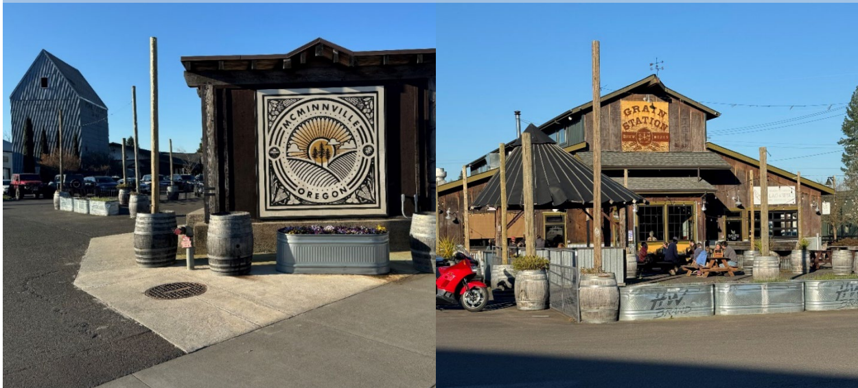
Grain Station Commercial Rehabilitation – Immediately to the south of the subject site
