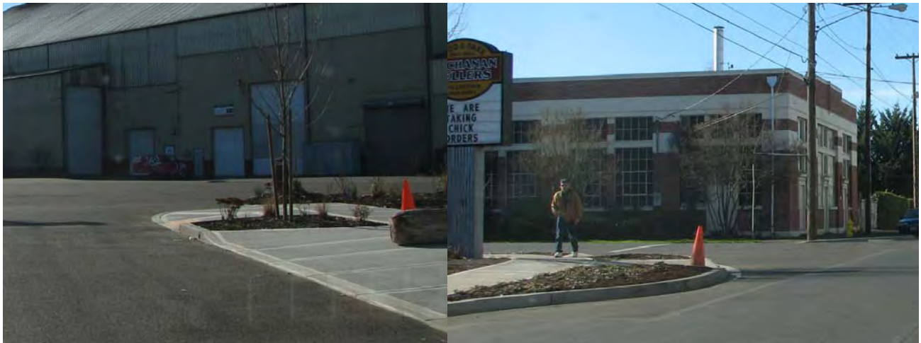
Granary District Sidewalk Improvements
