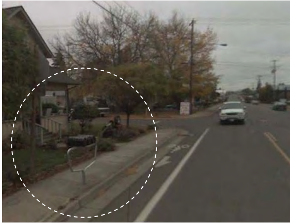
Sidewalk Obstructions on Lafayette Avenue
