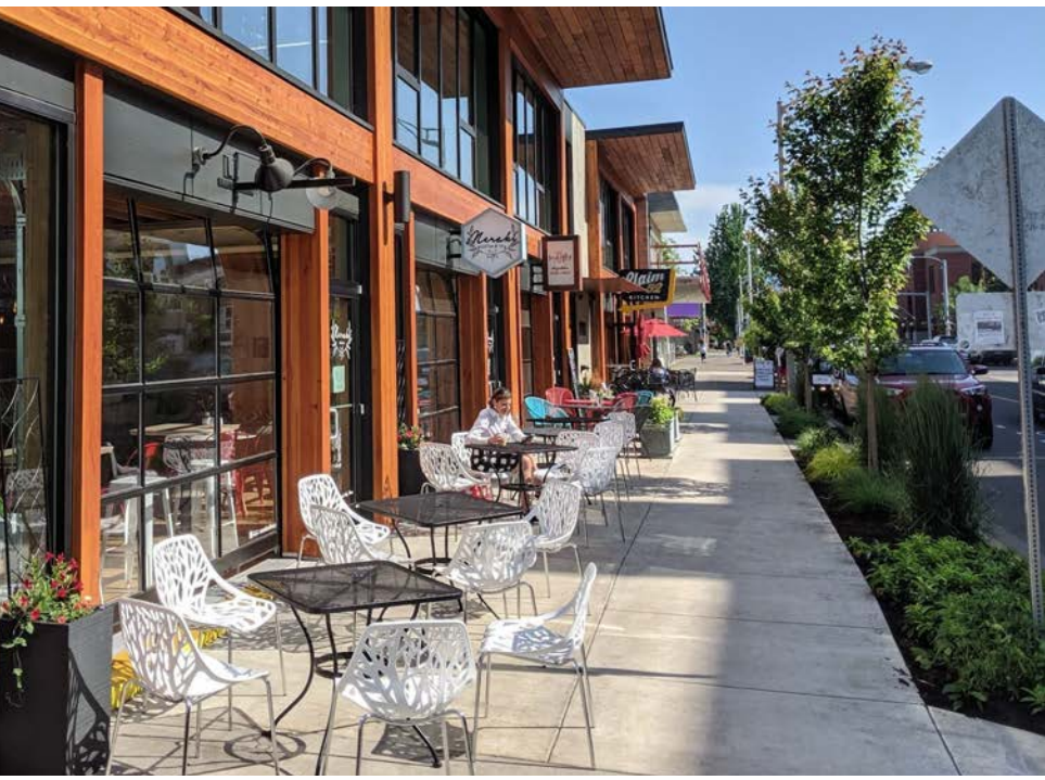
Outdoor seating and stormwater (Willamette St - Eugene, OR)
