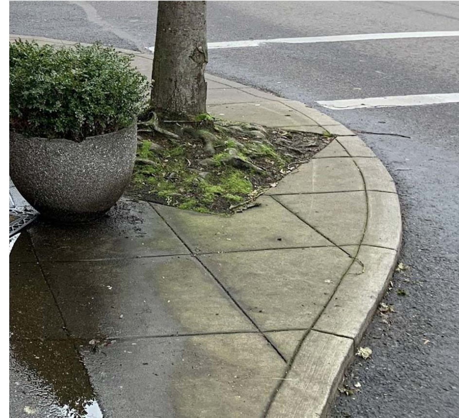
6" Concrete Curb (Existing)
