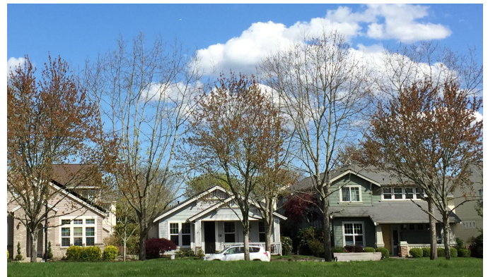
Usable side yard setback homes provide enough space for side yard patios. Adjacent homes were designed with high windows on the narrow setback side for added privacy.
