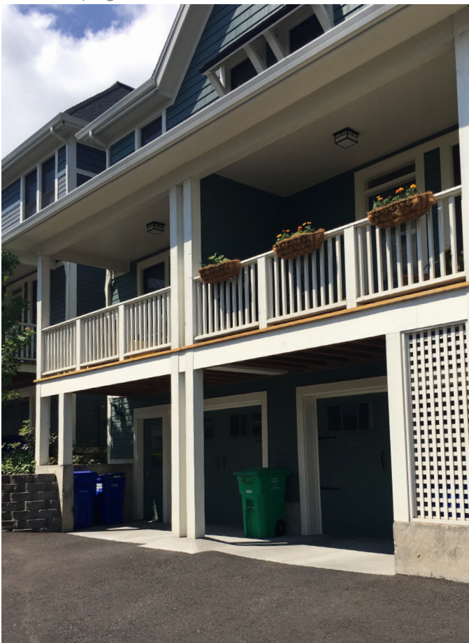
Garage doors set into an alcove created by a second story porch provides storage for trash receptacles and minimizes the prominence of the garage.
