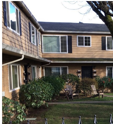
2-story courtyard apartment
