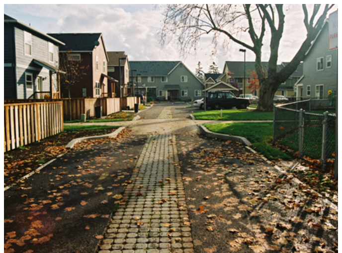
The curb physically and visually narrows the width of the alley. Permeable paving is built into the lowest point at the center to handle stormwater.
