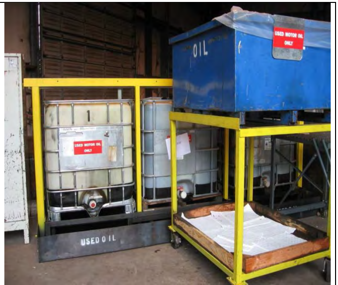
Used oil storage area inside the MRF building which has been upgraded and brought inside of the building.
