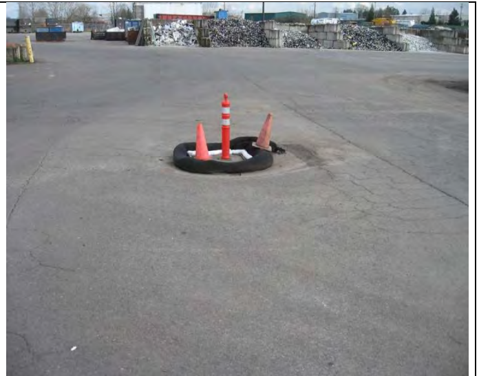
Glass storage bunkers in the background. The site is clean, swept, and all catch basins are clean and surrounded by various stormwater controls such as boom, filter socks and filter bags inside.
