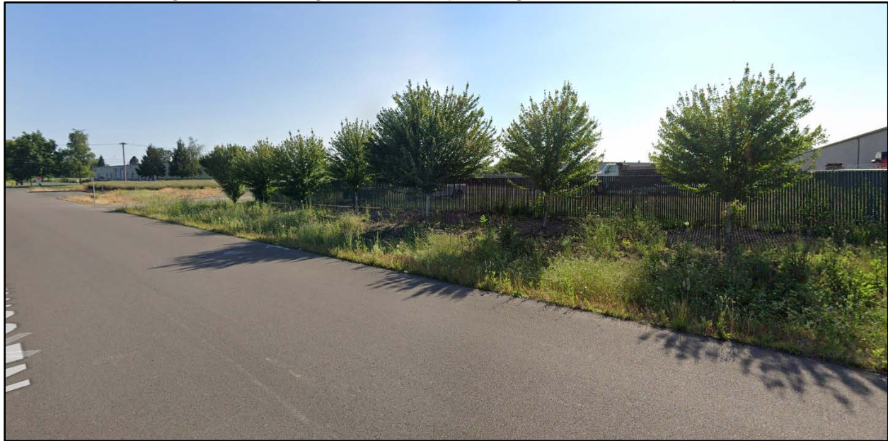
Figure 4: Existing Conditions (looking W from Colvin Court)
