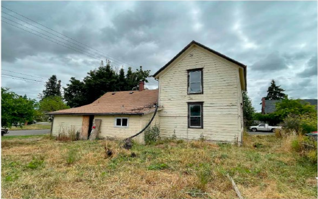
Figure 3: Photos of Current Exterior Conditions
