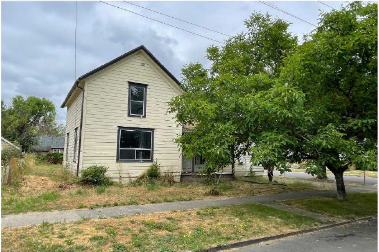
Figure 3: Photos of Current Exterior Conditions
