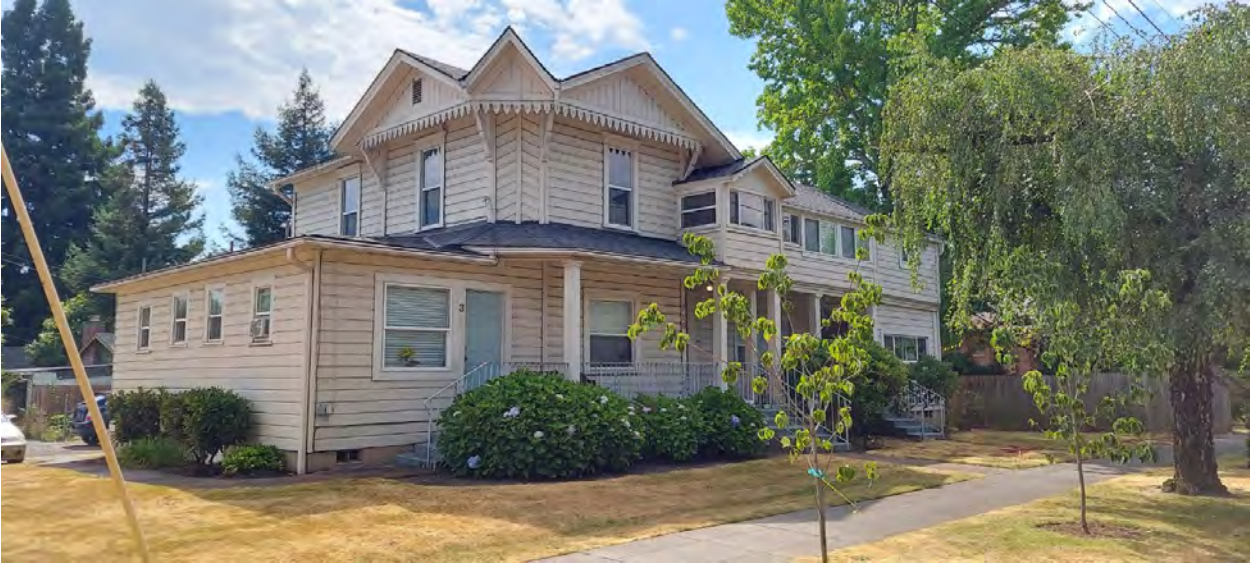
Figure 4: Photos of Current Exterior Conditions
