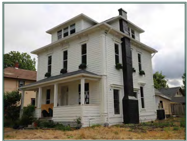
436 SE Baker Street (ca. 1870), Italianate house.
