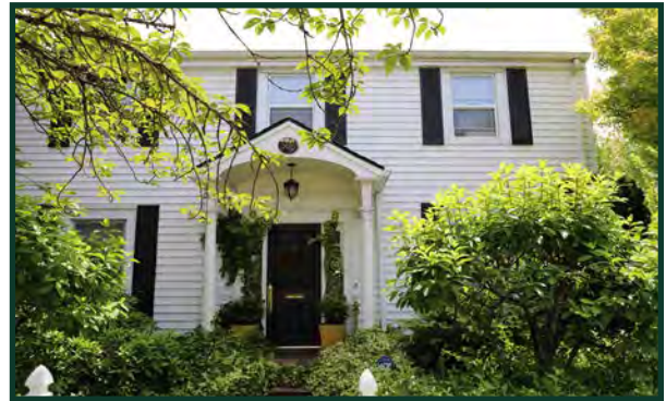
506 SE 1st Street (ca. 1930), a Colonial Revival example.
