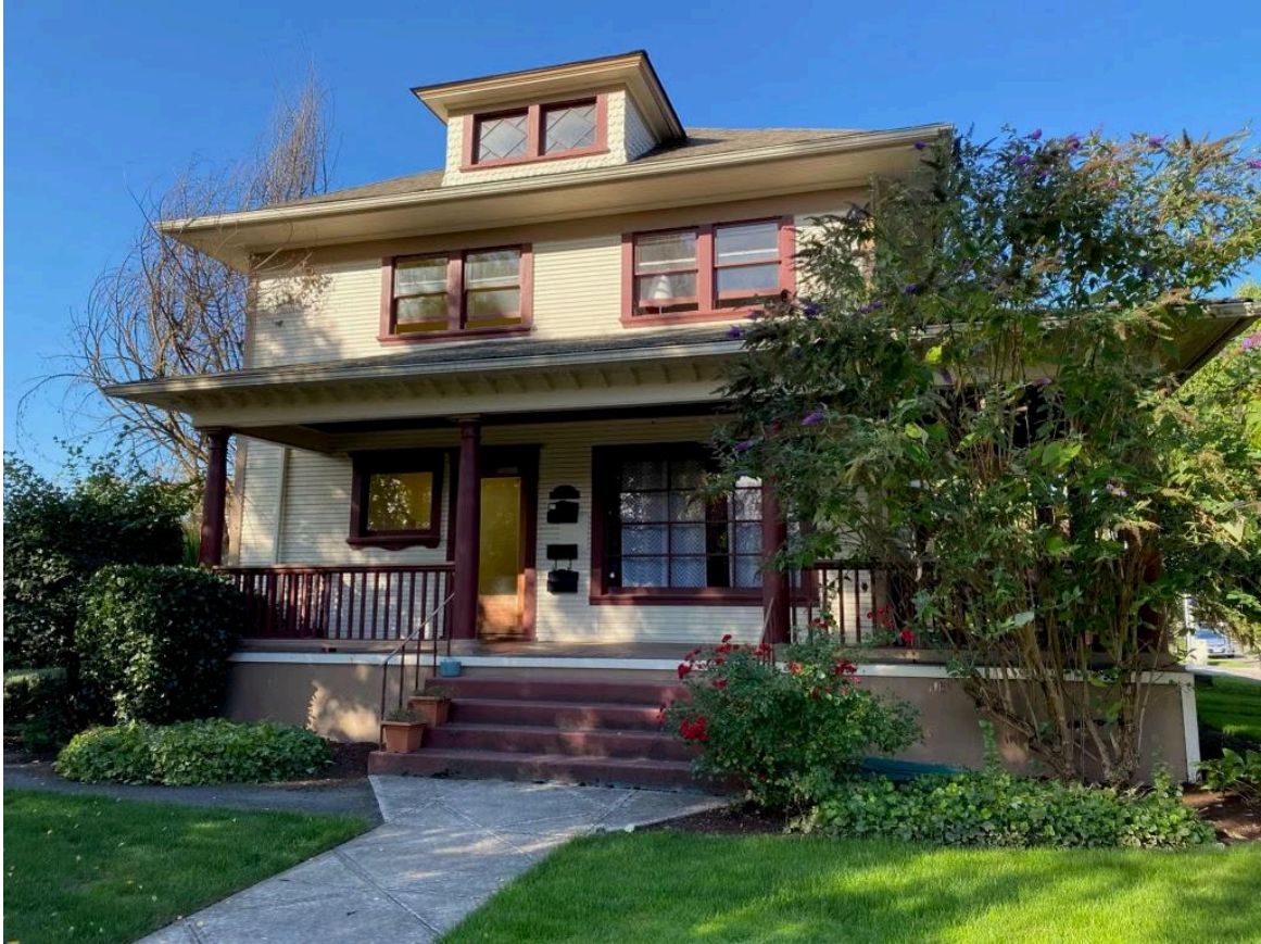
PHOTO 5: Second window added on the 2nd story, northeast corner of the house, probably by George Beeler in the 1940s when the house was subdivided into apartments. 1950's picture window has replaced original, single double-hung window.
