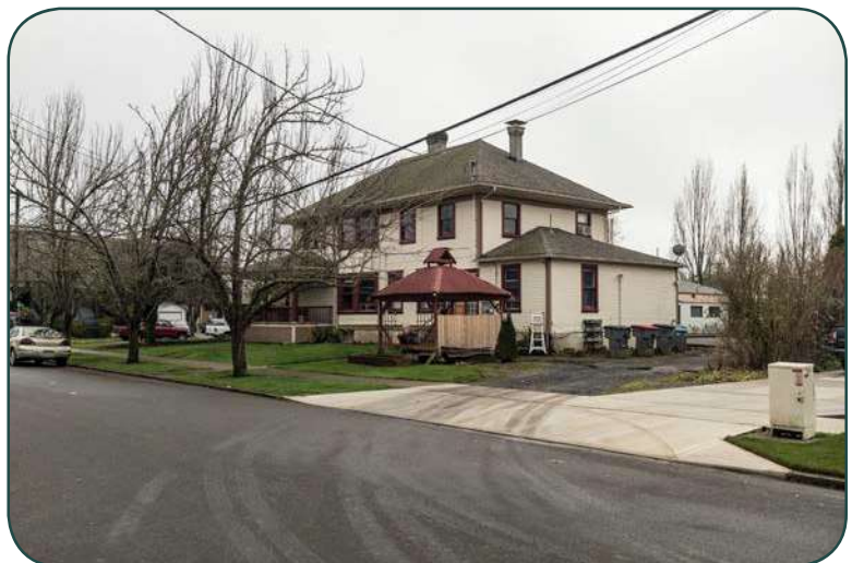
Side, north and rear west facades.
