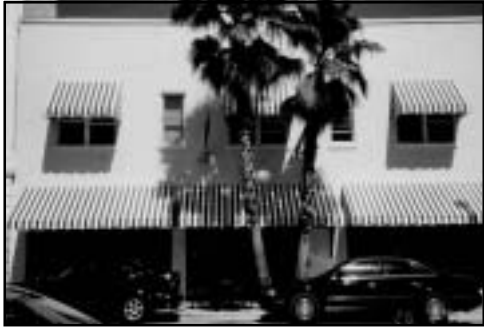
Rehabilitated 1920s commercial building.
