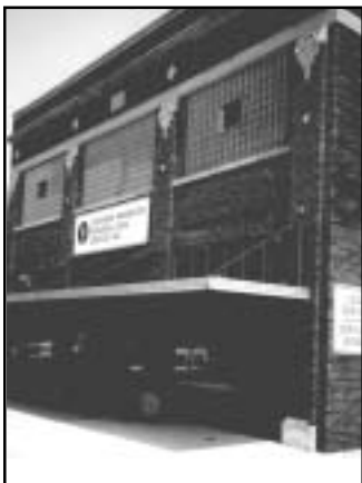
Rehabilitated dairy building.
