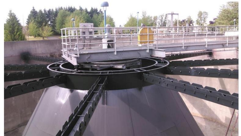
The City continued to invest in upgrades to the public sanitary sewer system in 2019. Work included recoating of tertiary clarifiers #1 & #2 and ATAD #3 at the Water Reclamation Facility.
