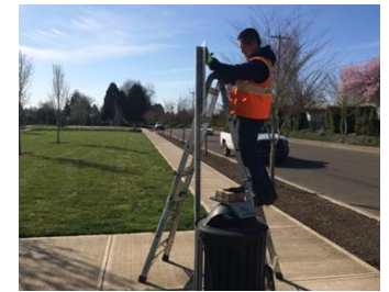
Carlos Ochoa – Street Crew – Installing new signage
