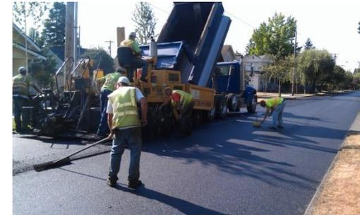
The City's annual pavement maintenance work in 2013 included approximately 1.6 miles of street overlays and the upgrade of 24 corner curb ramps to current accessibility standards.
