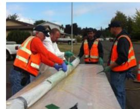
The Conveyance System team prepares a pipe patch for a trenchless sewer line repair.
