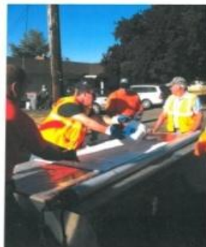
The Conveyance team prepares a pipe patch using a new lining system instituted in 2011. With the “Logiball” repair system small sections of pipe can be rehabilitated using in-house staff and resources.
