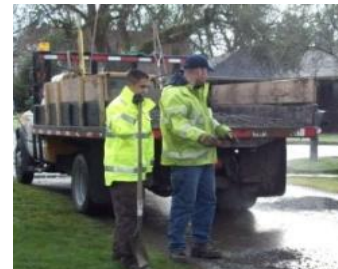
City gravel street work.
