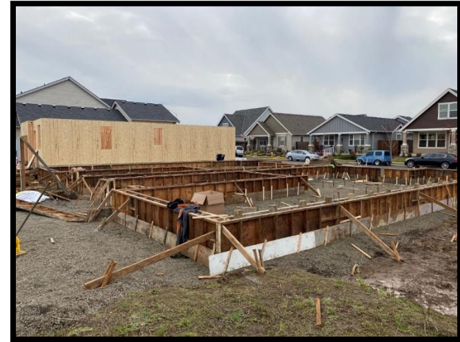
Small Lot, Small Home Subdivision Foundations
