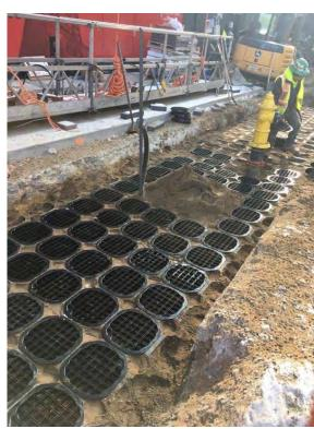
**Soil Cells** can promote root growth below paving by providing trees more space and uncompacted soil
