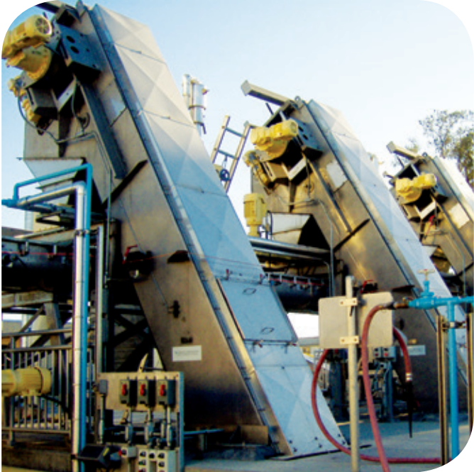
Retrofitted screen with perforated plate screening surface and solids-carrying shelf.
