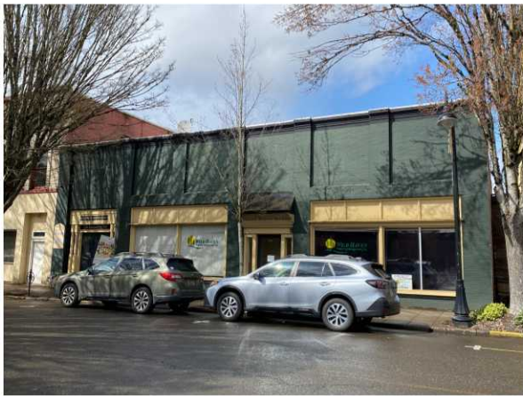
Front Half of the Bennette Building - 619 NE 3rd St.
