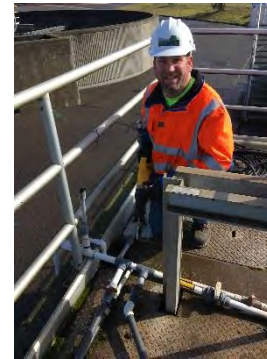
Roy Carter, Mechanic, works on the tertiary chemical distribution system.
