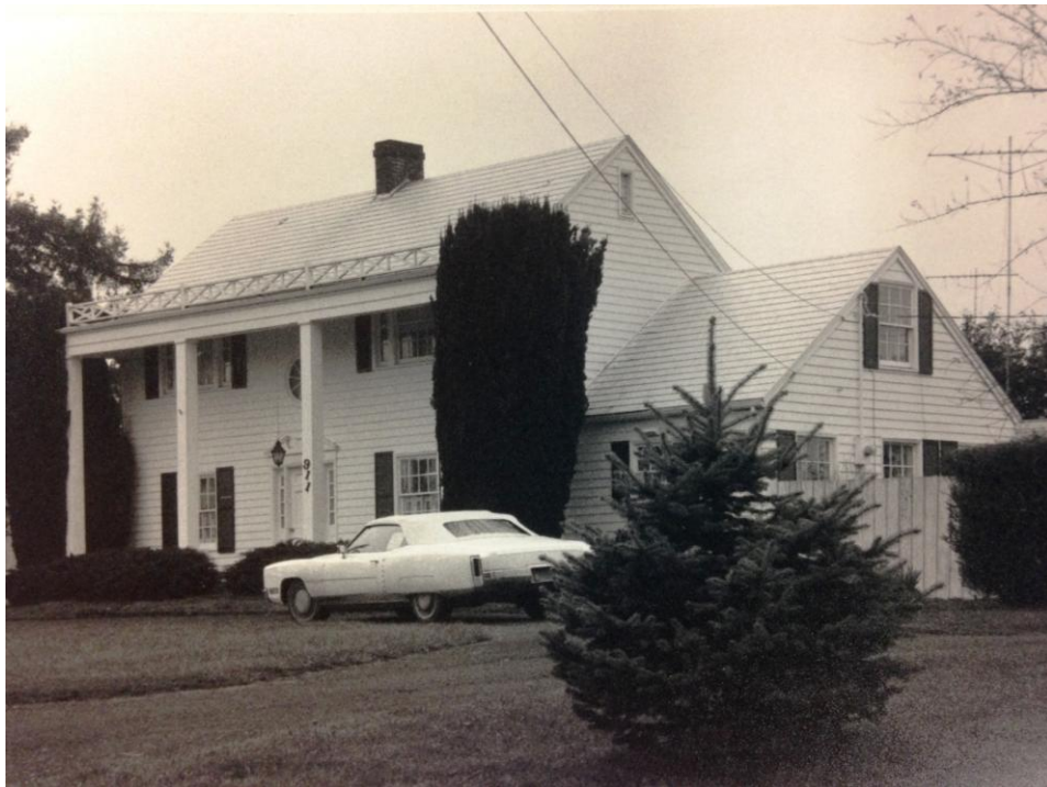
Original 1983 Survey Photo
