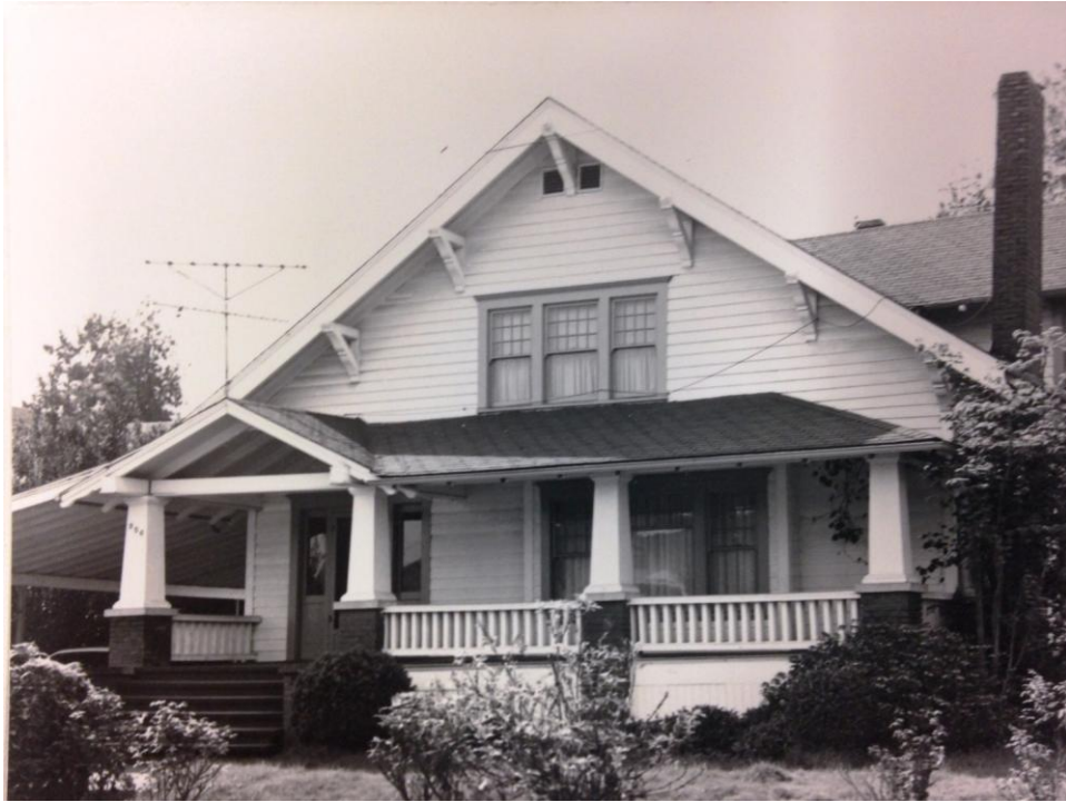
Original 1983 Survey Photo
