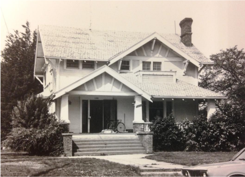
Original 1983 Survey Photo
