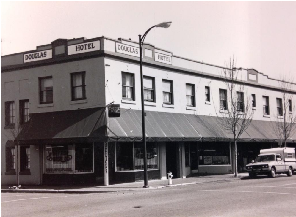
Original 1983 Survey Photo
