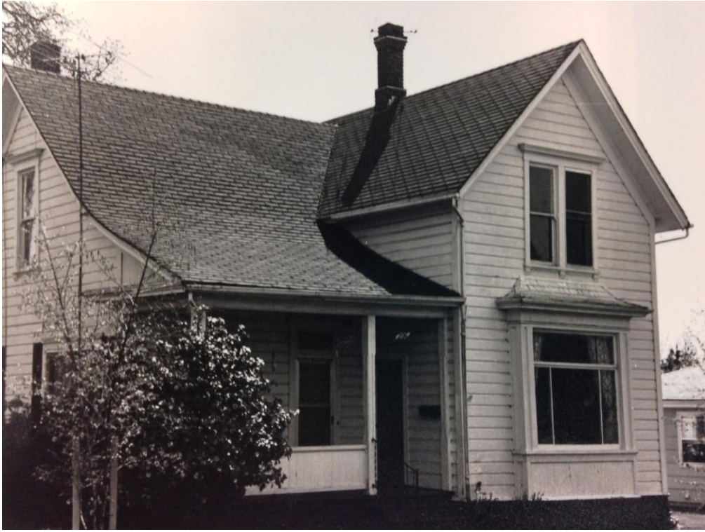
Original 1983 Survey Photo
