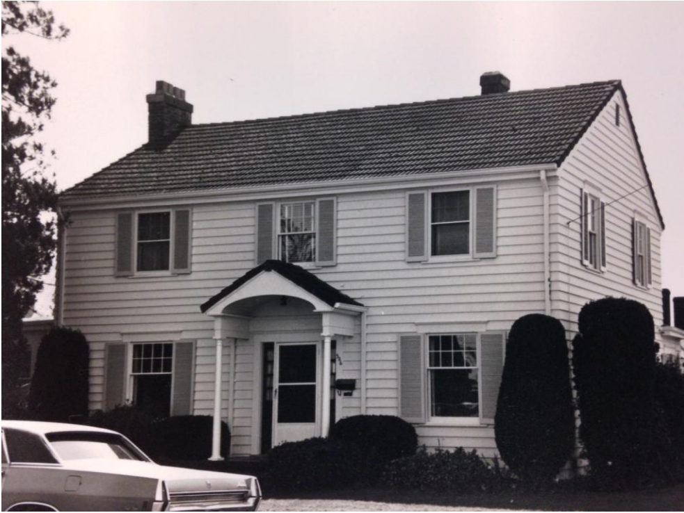
Original 1983 Survey Photo
