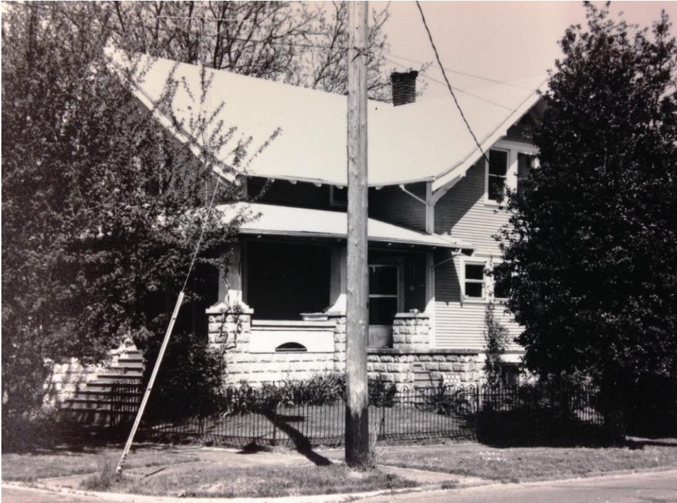
Original 1983 Survey Photo
