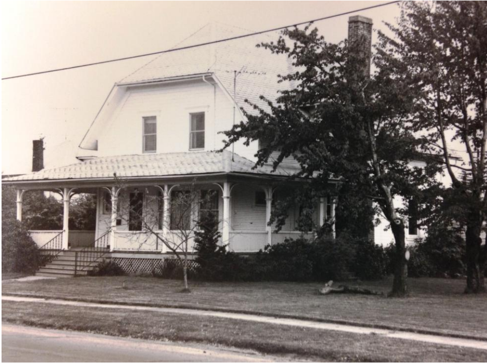
Original 1983 Survey Photo
