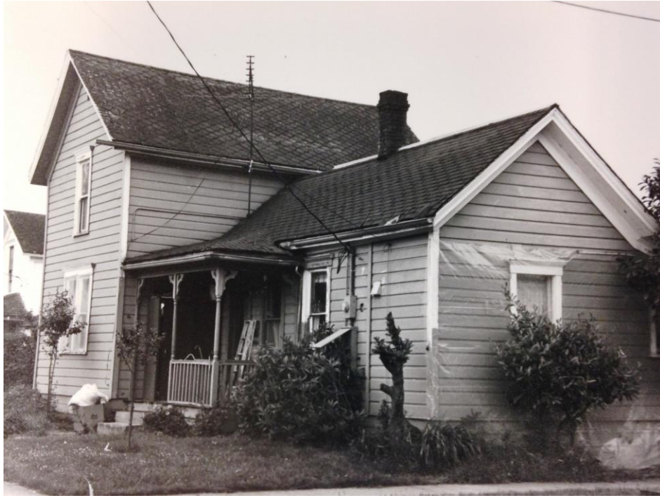
Original 1983 Survey Photo
