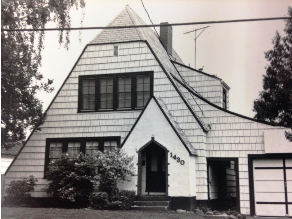
Original 1983 Survey Photo
