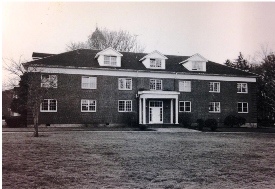
Original 1983 Survey Photo
