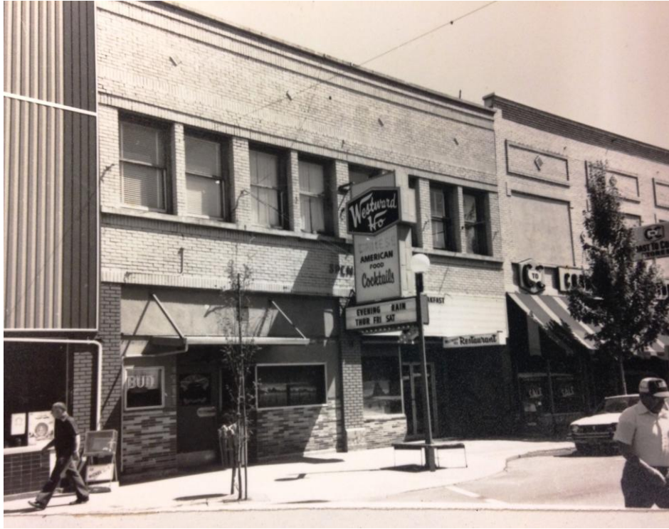
Original 1983 Survey Photo
