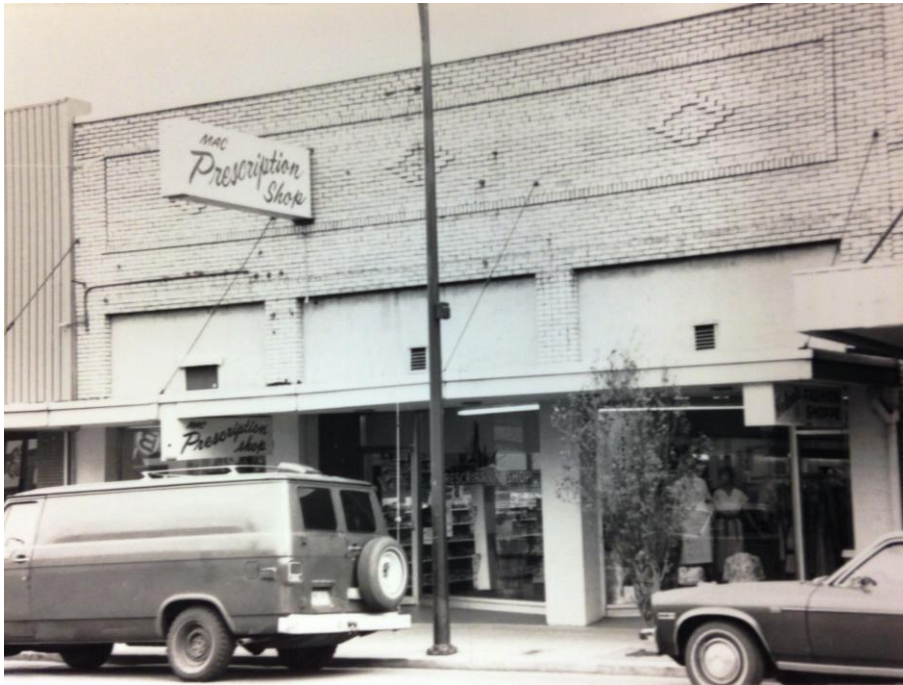
Original 1983 Survey Photo
