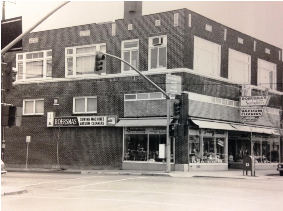
Original 1983 Survey Photo
