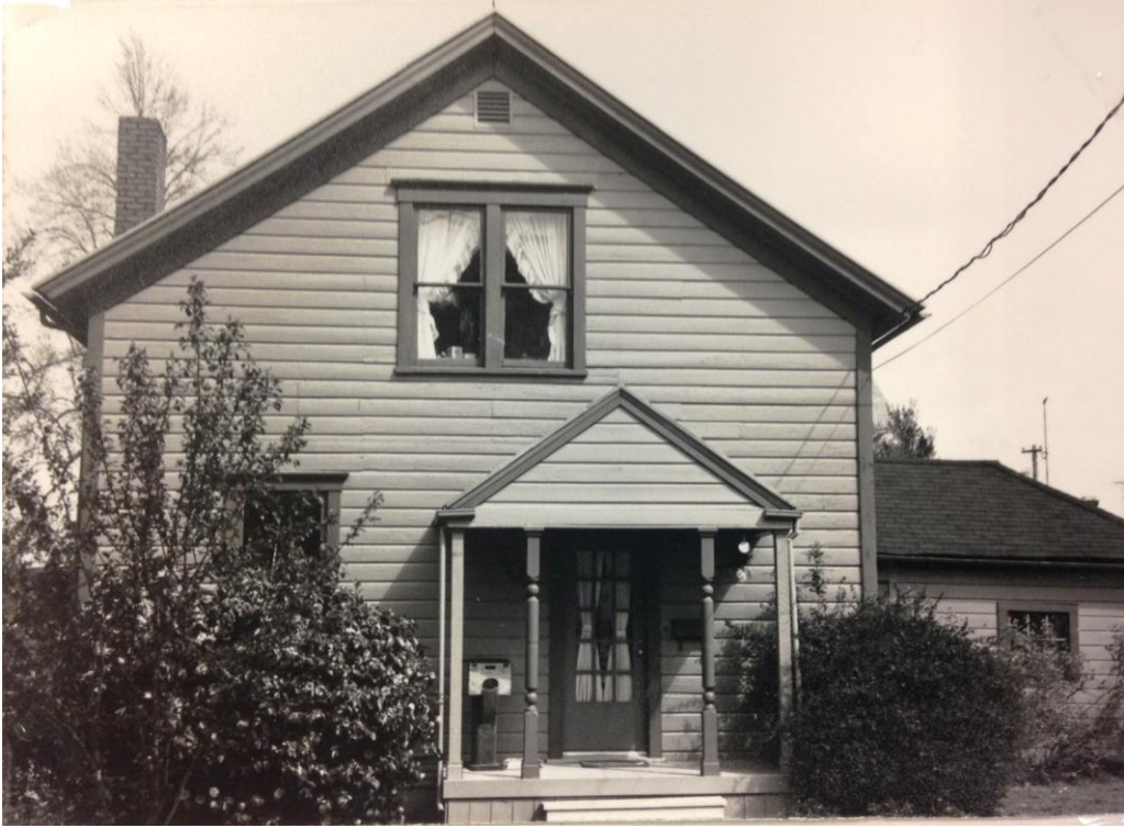
Original 1983 Survey Photo
