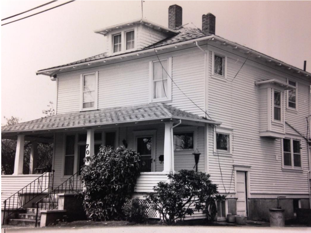
Original 1983 Survey Photo
