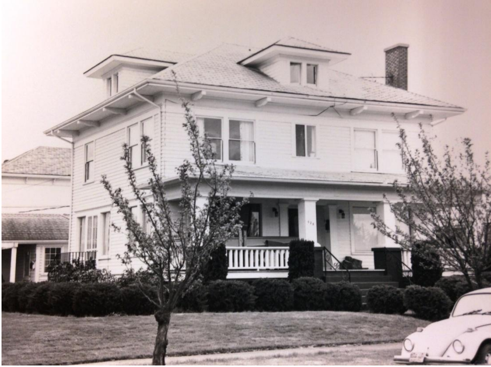
Original 1983 Survey Photo
