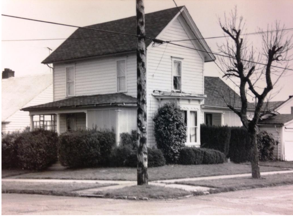
Original 1983 Survey Photo
