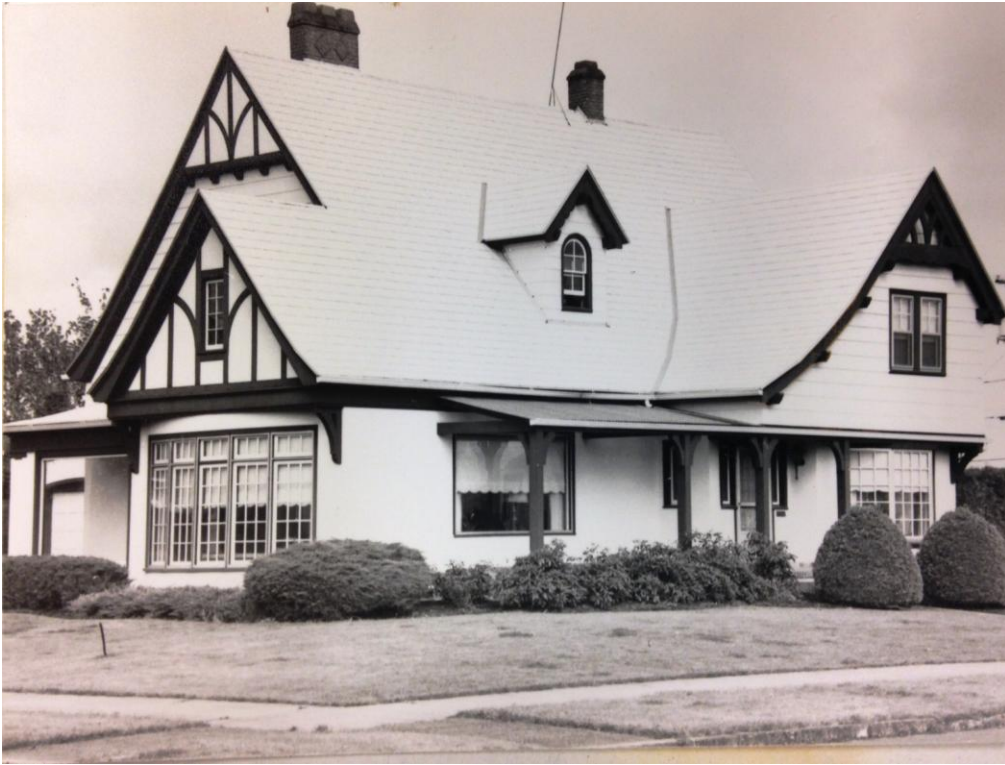
Original 1983 Survey Photo
