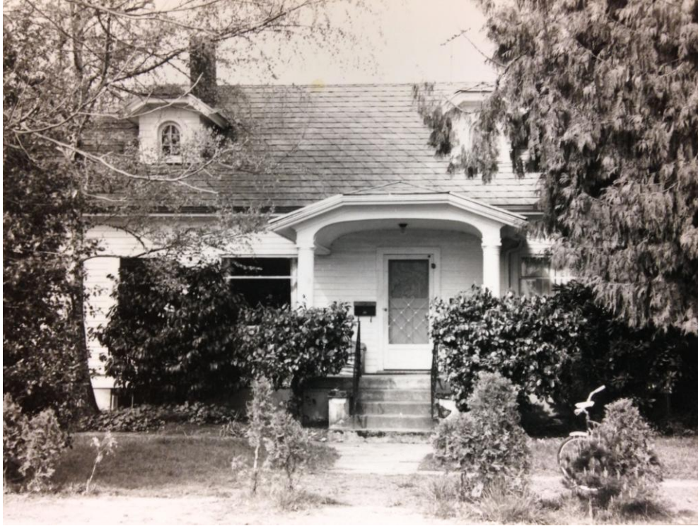
Original 1983 Survey Photo
