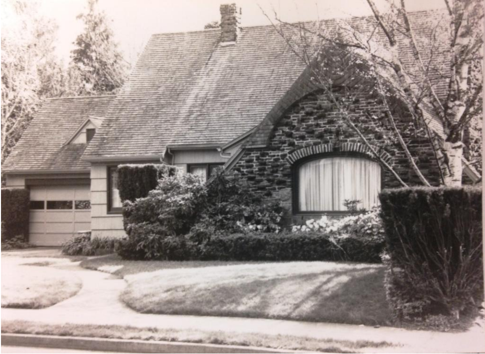
Original 1983 Survey Photo
