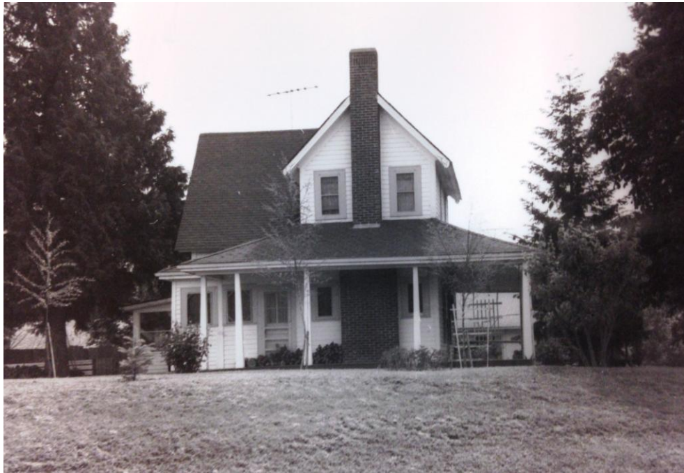
Original 1983 Survey Photo
