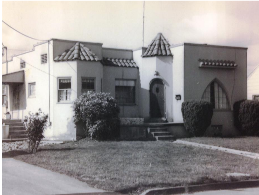
Original 1983 Survey Photo
