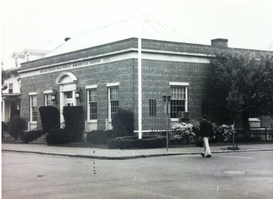
Original 1983 Survey Photo
