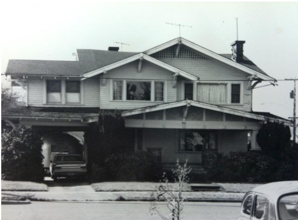
Original 1983 Survey Photo
