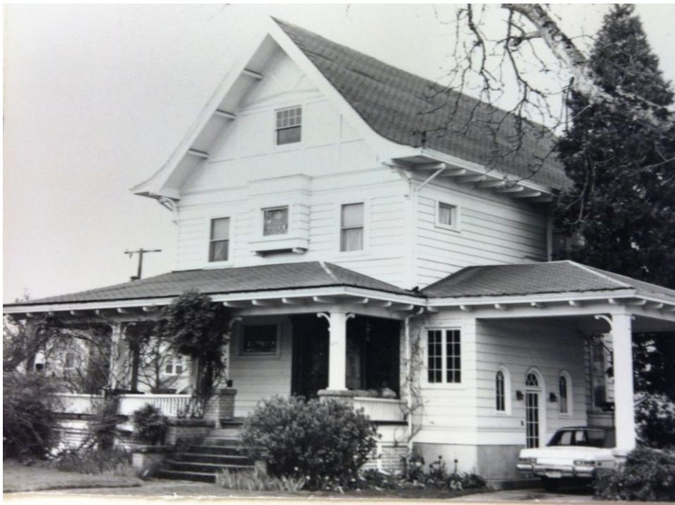
Original 1983 Survey Photo
