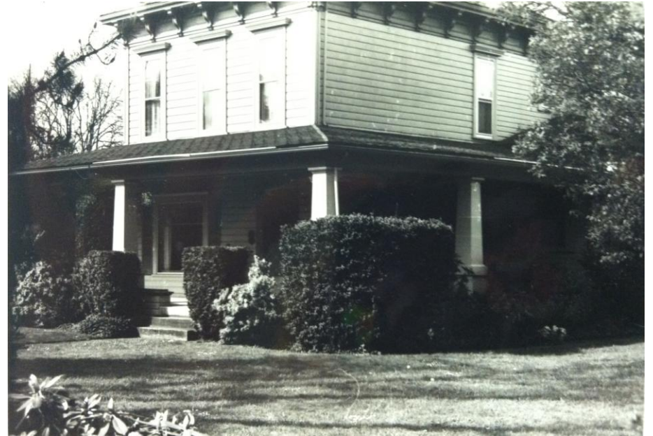
Original 1983 Survey Photo
