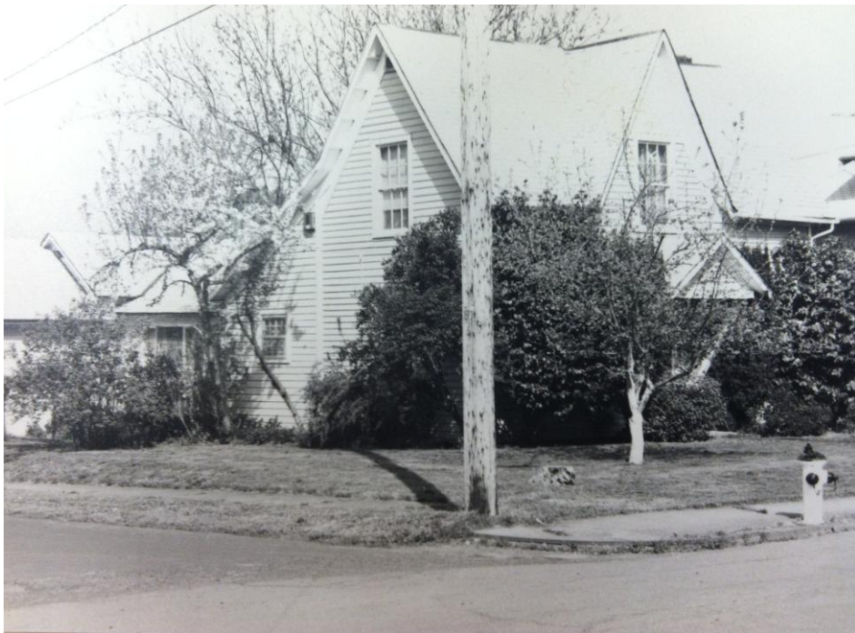
Original 1983 Survey Photo
