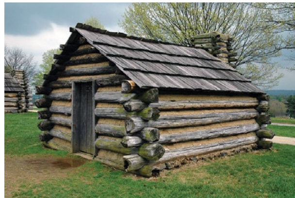
[7] The Muhlenberg Brigade Huts are reconstructions of nine log huts erected in 1777 at Valley Forge during the Revolutionary War. They have been reconstructed on the historic road with logs cut with modern power tools and finished with cement, unlike the original logs which were hand hewn and finished with traditional chinking. Photo: Rdsmith4 at Wikimedia Commons.
