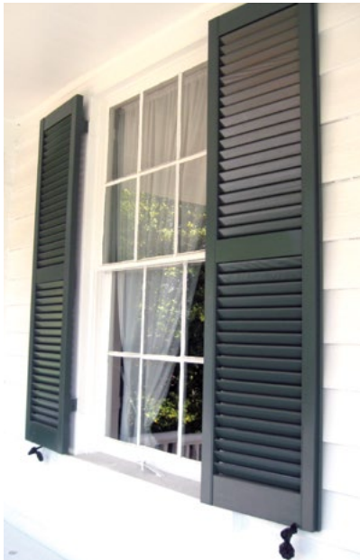
[9] Historic window and shutter hardware such as that shown here should be retained and repaired in a restoration project.
